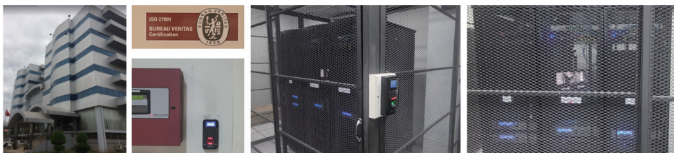
Figure 5. PKI Center in LANIC Data Center
