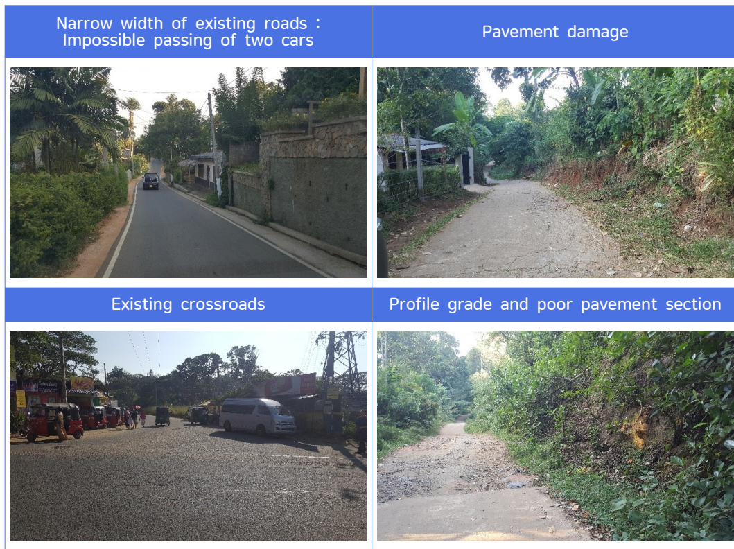
Figure IV-7 | Current situation of road in Kandy
