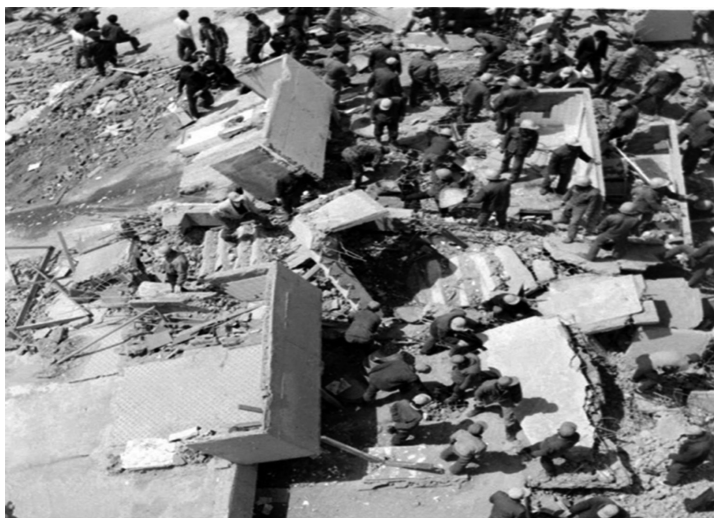
[Figure 2-9] Collapsed Citizen's Apartment (Wawoo Apt.), Seoul, 1970
