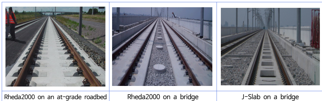
Figure 65 | Concrete Tracks Laid in At-grade & Bridge Sections in Foreign Countries
