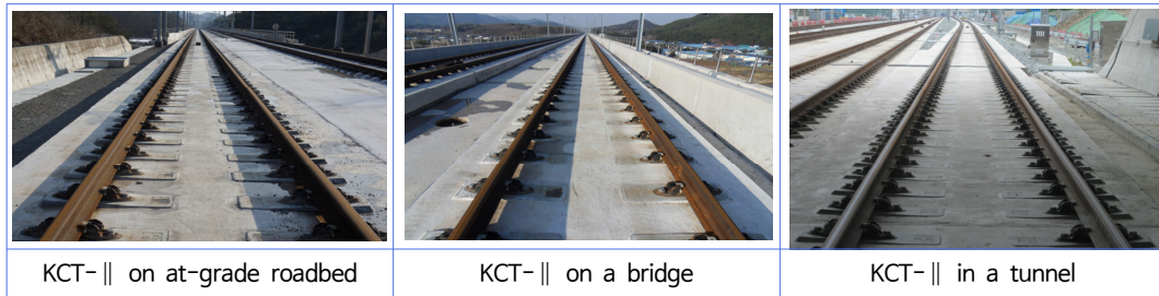
Figure 64 | Concrete Tracks in Gyeongbu HSR Phase 2
