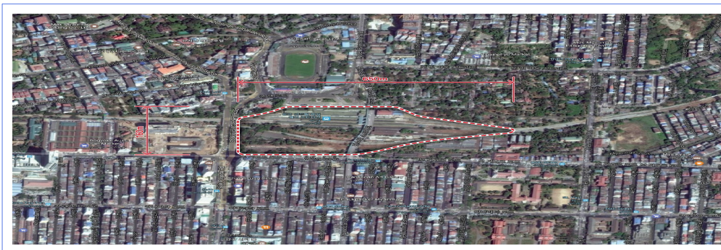
Figure 40 | Present Situation of the Existing Yangon Station
